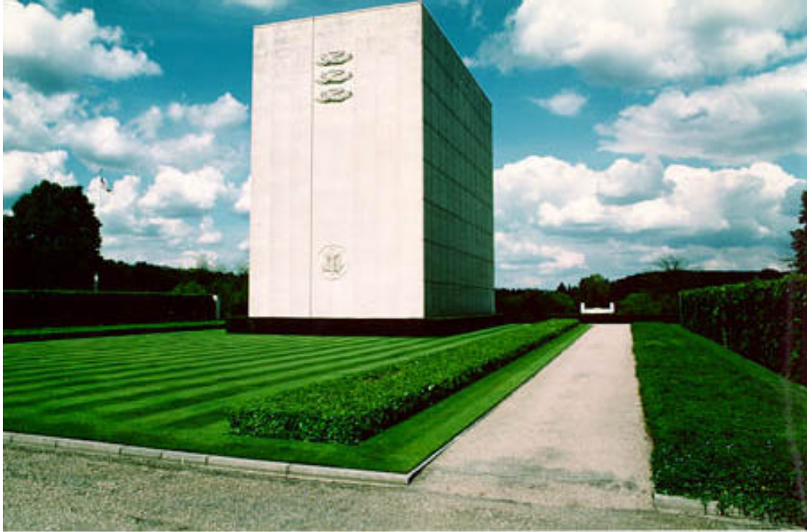
West Facade of Memorial
